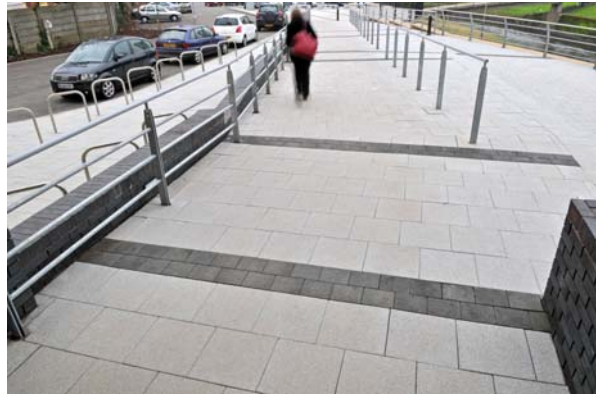
To building entrances and footpaths: Granite concrete paving flags, preferably permeable: e.g. Mayfair by Tobermore (image copyright Tobermore)
