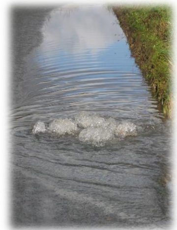
Water exceeding drainage system via a manhole (© JBA Consulting)
