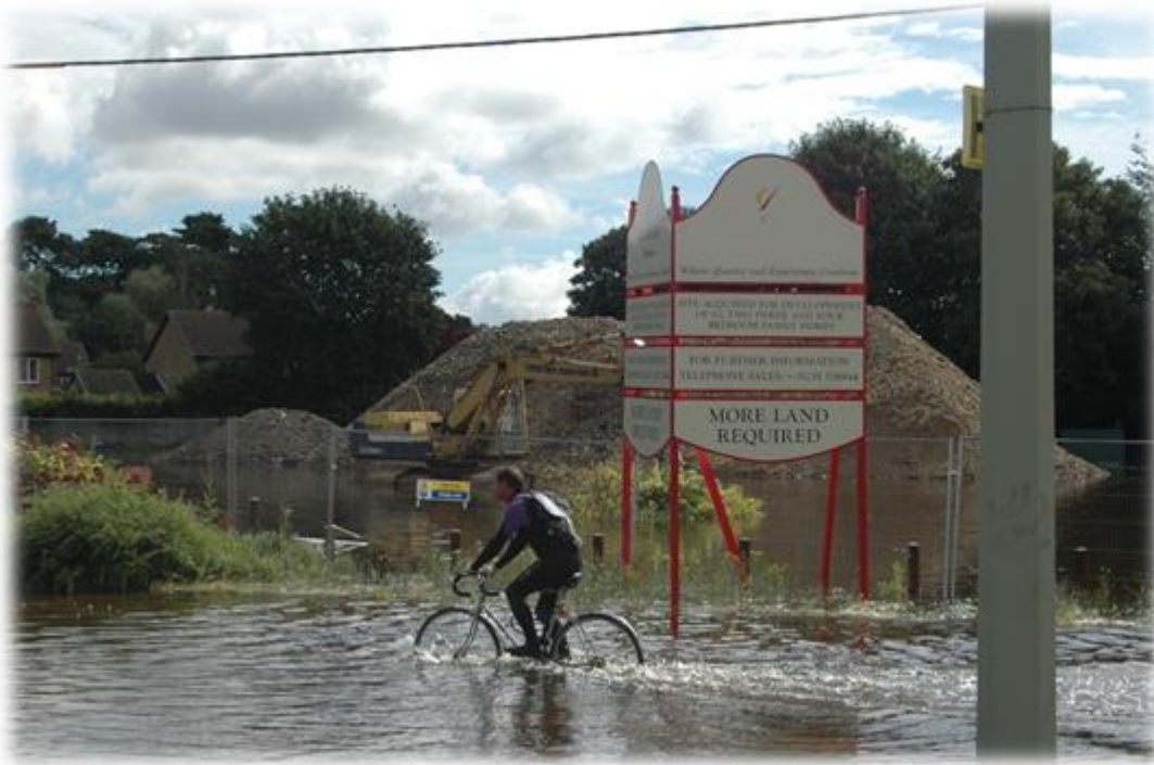
Flooded development site (© JBA Consulting)
